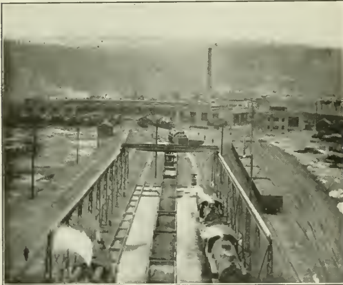
Cinder Pits and Roundhouse With Machine Shop and Old Roundhouse on the Right.
